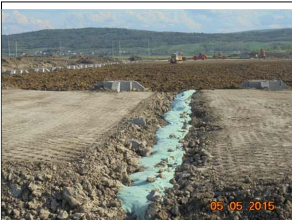
Drenuri transversale - Hala Mecanica..
