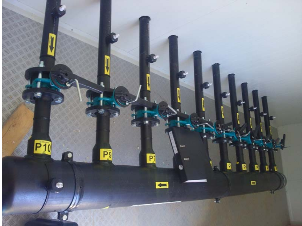
Container regularizare debit biogaz – detalii
