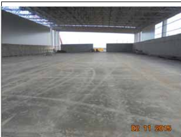
Pardoseala, Hala Tratare Biologica..
