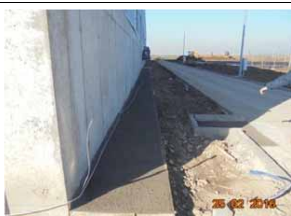
Turnat trotuar, fatada principala, Hala Tratate Mecanica.
