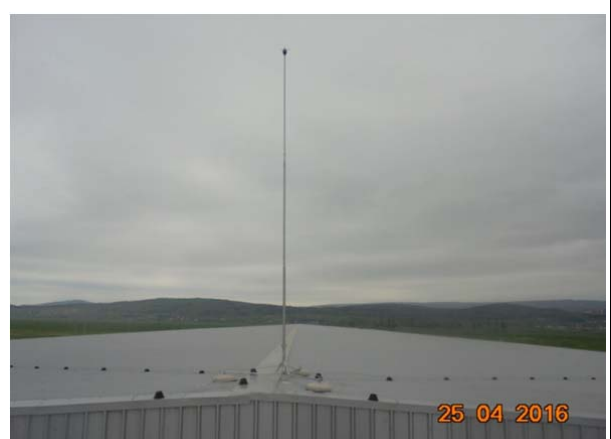
Montat paratraznet, Hala Tratate Mecano-Biologica
